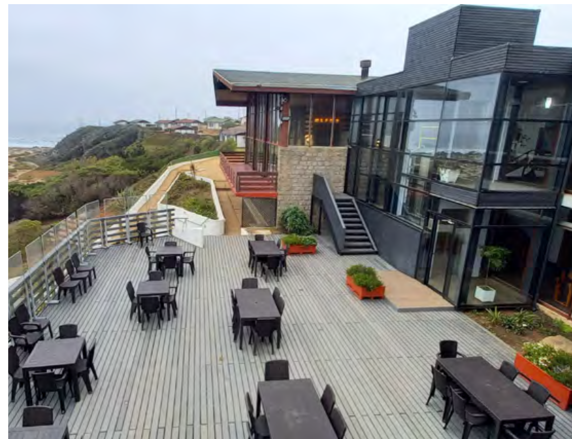
At the CBC beach resort, the terraces and stairways are made of recycled plastic wood.
