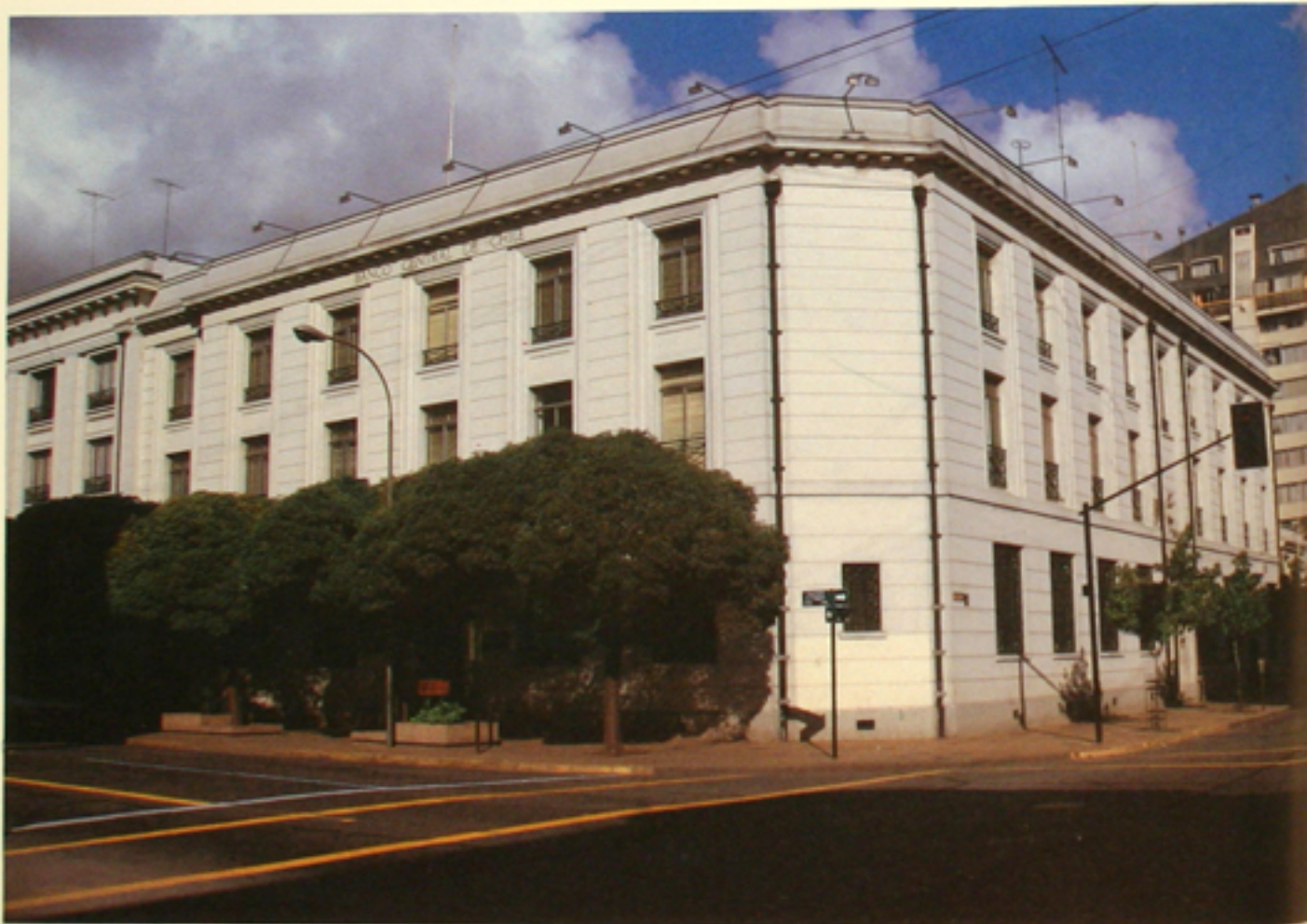
BANCO CENTRAL DE CHILE Branch in Concepción
